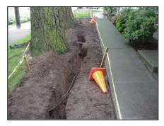
Excavation of mini soakage trench along south side of the property; 2002
