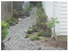
The trench filled with gravel and planted along the edges; 2002
