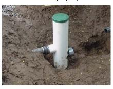
One of 13 cleanouts installed where subsurface downspout extensions enter the trenches and basins
