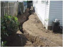
Excavation of mini soakage trench along SE edge of property; 2002
