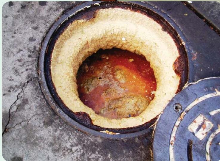
Ideally, under Cut Through the FOG all Portland food service establishments would plumb all FOG-generating fixtures to a single large capacity gravity grease interceptor, enlist help from a reputable pumping company to handle cleaning, maintenance
