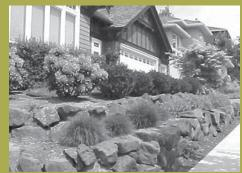
Use tiered planters to stablize slopes, protect against erosion, and reduce sediment transport.
