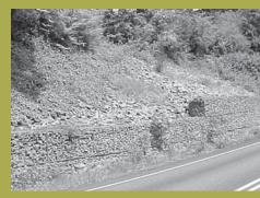
Highly erosive or unstable soils may require reinforced soil retaining systems or armoring.
