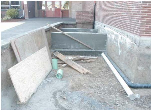
**Figure 3: Monitoring, flow-through, and infiltration cells of stormwater planter retrofit (from back to front of photo)**
