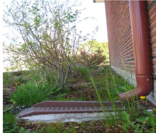
**Figure 5: Disconnected downspouts in stormwater planter**
