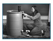
2 Overflow: Drill a hole near the top of the barrel to accommodate an overflow pipe that is at least 2 inches in diameter. If the overflow pipe elbow seals and seats securely, it can be threaded directly into the barrel opening. If not, it should be secured with washers on both sides of the barrel and a nut on the inside. Use Teflon tape around the threads and a bead of silicon caulking around the opening to ensure a tight seal.
