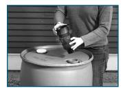
1 Inlet: Create an opening with fine screening through which the rain barrel will collect water from the downspout elbow. This can be a single screened opening large enough to accommodate the downspout elbow (as shown in the photo), or a series of smaller screened openings directly in the top of the barrel.
