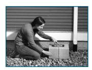
**3** Foundation: Create a raised, stable, level base (like concrete blocks) for the rain barrel to sit on. You might want to test stability by filling the rain barrel with water before attaching to your structure. A full rain barrel is very heavy and tipping is a risk if it's unsecured or on an uneven surface.
