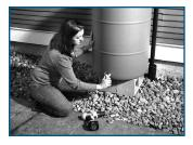
5 Outlet: Drill a hole near the bottom of the empty barrel to attach the drain spigot. If the spigot seals and seats securely, it can be threaded directly into the barrel opening. If not, it should be secured with washers on both sides of the barrel and a nut on the inside. Use Teflon tape around the threads and a bead of silicon caulking around the opening to ensure a tight seal.
