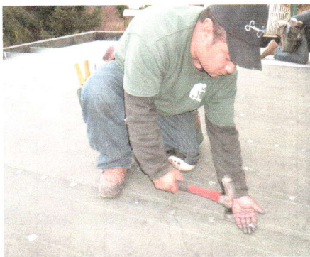
Installing membrane
