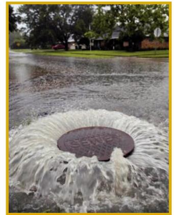
**Grease clogged sewer pipe overflowing into street.**
