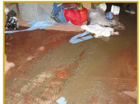
**Grease clogged sewer pipe overflows into residential basement.**
