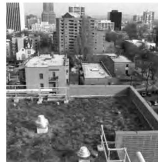
Ecoroof systems capture runoff before it flows to sewer system.
