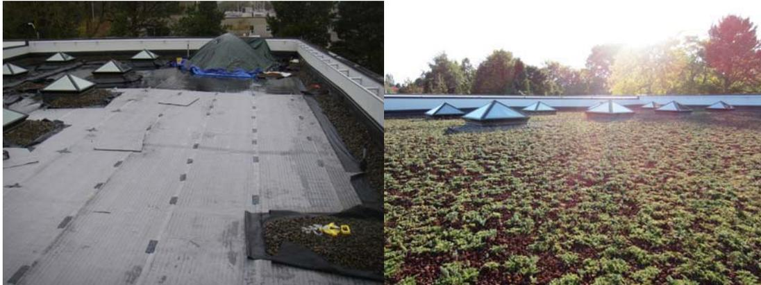
A one inch layer of red cinder was placed over the cuttings as a mulch to retain summer moisture, eliminating soil erosion and the need for an irrigation system. The photo above right shows the ecoroof in fall after the first summer with no irrigation. River rock paths facilitate maintenance access to the skylights and add diversity.
