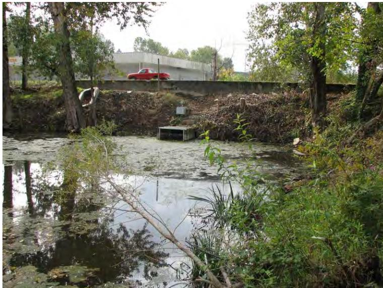
Undersized culvert at NE 33<sup>rd</sup> Drive and Buffalo Slough to be replaced in 2013.
