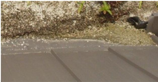
On the front porch roof, moderate rains caused a stream of water to overflow the lower edge of the "side channel" where some of the metal house roof meets the edge of the ecoroof perpendicular to the ecoroof slope. We built up a higher "dam" with metal caulked to the existing edge, which now allows excess water to enter a drainpipe running from that spot towards the gutter. The picture on the left shows eroded soil piled up against the original, shallow edge at the far right.
