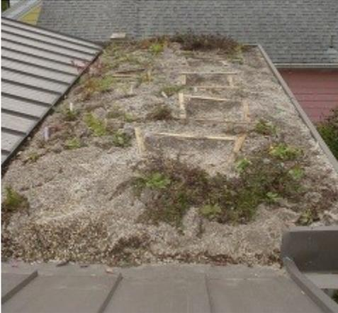
136.5 ft<sup>2</sup> (7' 3" x 18' 10"): The front porch roof slopes north with about 1/12 pitch. It receives full sun year round. It holds 8" of intensive B-4 soil mix.
