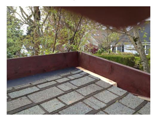
Then a grid of 1x4s was put in place under the  $\frac{3}{4}$ " plywood sheeting and an 8' galvanized drip vent was inserted along the low end of the slope.
