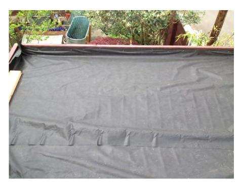
Two 2x4s were added to divide the eco-roof into three segments. This was to minimize slippage of soil and plants.
