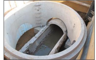
*Pre-constructed manhole segments to replace old manhole on the 120-year-old sewer*
