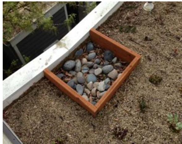
2x8x12' Pressure treated board and river rock for scupper dams
