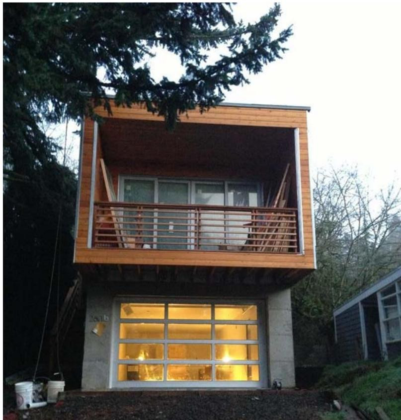
Structurally there was negligible impact of the added weight of the green roof as my 16' roof joists already needed to be oversized to 2x12's in order to accommodate the required insulation. The only change was that some of the shear walls were beefed up to deal with the addition potential seismic forces.
