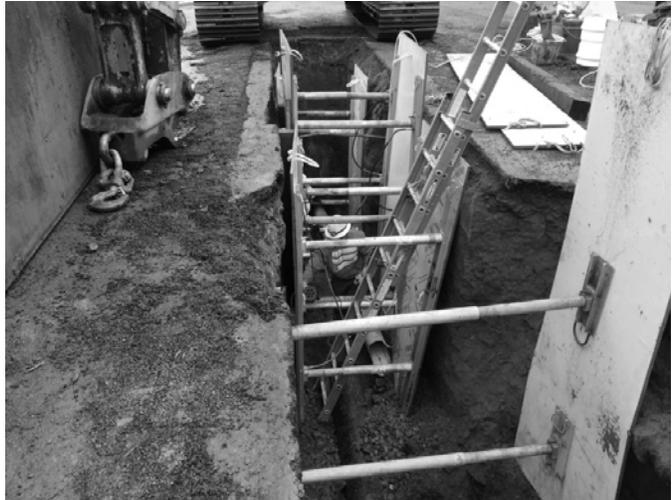
Crews connect the new sewer to a manhole.
