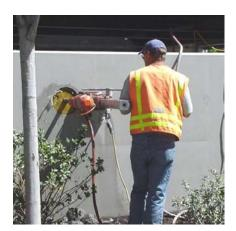
Coring through concrete wall for stormdrain and scupper, 2002
