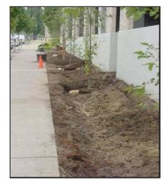
Excavated easts ide infiltration planter under construction 2001 (prior to curbs)
