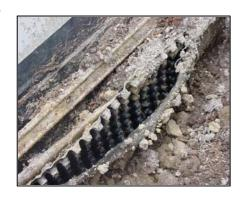
Foundation protection system: impervious seal and drainage panel
