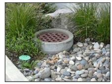
Overflow standpipe at southern end of infiltration basins
