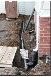
Installation of rain drains within two feet of fourndation; October 2002
