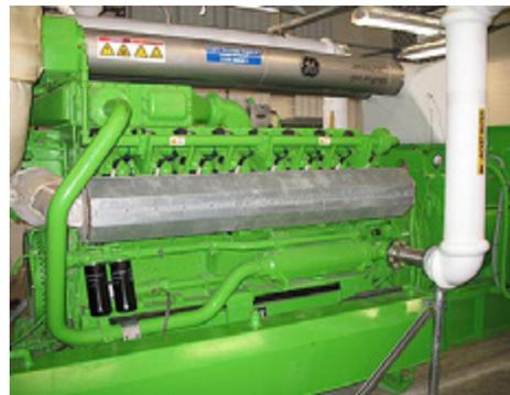
*These engine generators use biogas to produce about 40 percent of the CBWTP’s electricity needs.*
