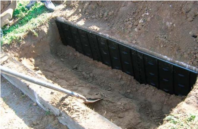
*DeepRoot barriers are made of injection molded polypropylene and are .080" thick.*
