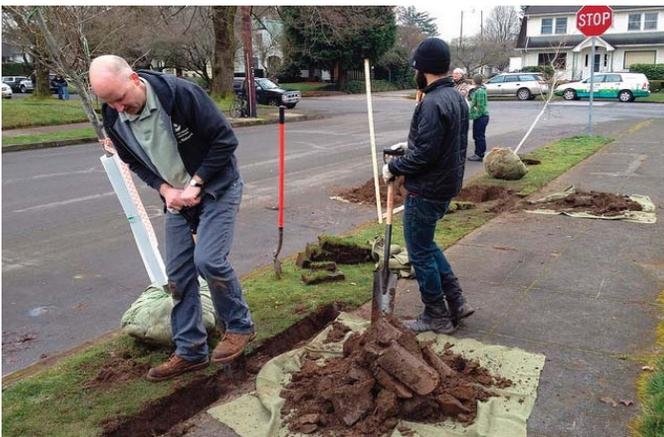
UF staffer Karl Dawson (left) digs a trench where a rigid root barrier will be installed flush with the sidewalk.
