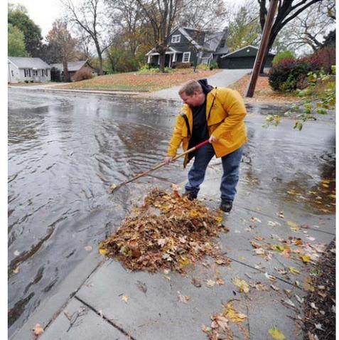
**Stand on the curb, rake debris off top of the storm grate, and dispose of debris properly.**
