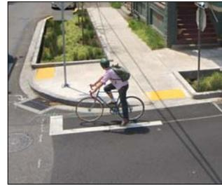
Curb extensions reduce delay by shortening the crossing distance for cyclists and pedestrians and creating more acceptable gaps in the passing traffic for safe crossings.
