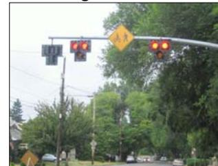
Hybrid pedestrian/bicycle signals are a new type of pedestrian or bicycle activated signal that provides a 'red and yellow' indication when needed, but dwells in dark (no green) when not needed, minimizing delay for traffic.
