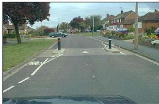
Pinch points reduce the roadway from two travel lanes to one at select locations, requiring 'courtesy queuing' when cars pass each other. Some on-street parking removal is required.
