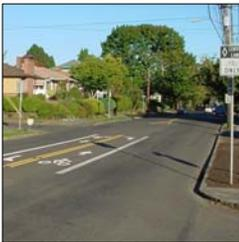
Off-set turn lanes create a safe place for cyclists needing to make left turns at off-set intersections. On-street parking removal may be required.
