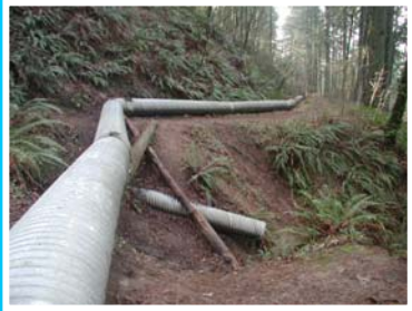
Water Bureau crews realigned stormwater drain pipes off the Holgate Trail.
