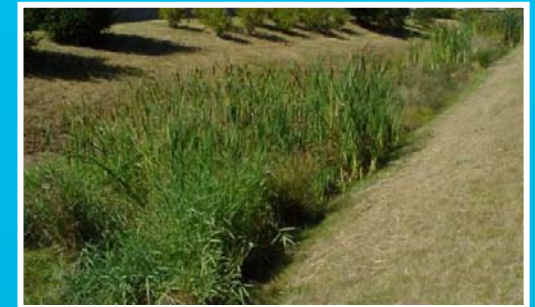
A 2005 drainage study that included local citizen involvement proposed bioswales as an alternative to concrete drain ditches for the new reservoir.
