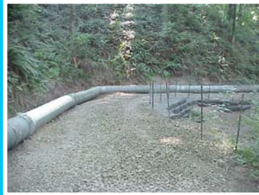
Water Bureau crews realigned stormwater drain pipes off the Holgate Trail.
