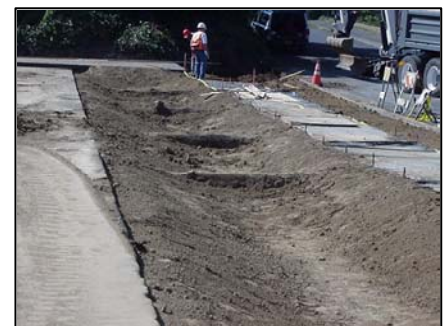
Installation of log check dams; August 2002
