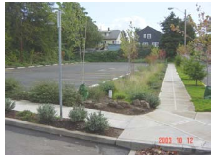
The parking lot and swale; October 2003
