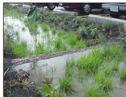
Log checkdam holds water back following a storm; November 2002
