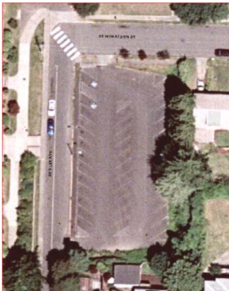
Aerial view of the Glencoe parking lot before retrofit; 2002
