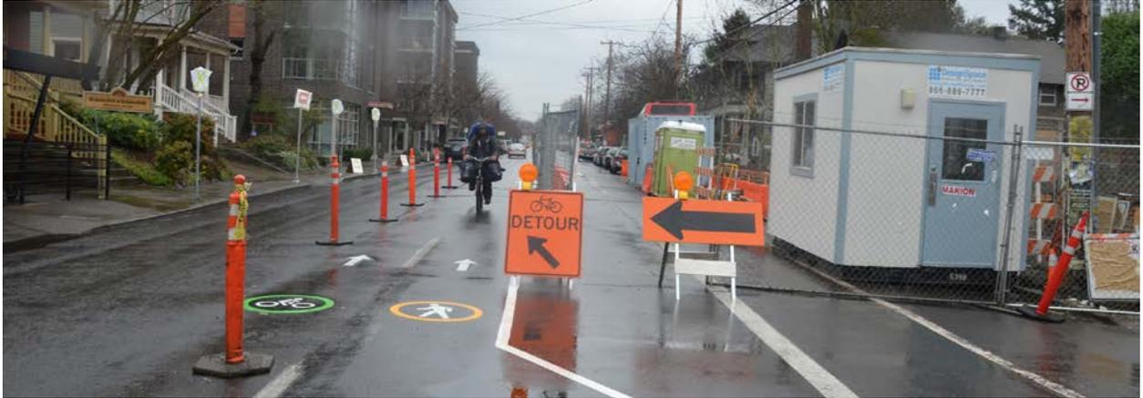
Another example of a high-quality detour is located on N Willamette Blvd. Where a retaining wall construction project closed the southern half of the roadway and forced westbound auto traffic to detour, the work zone maintained the eastbound bicycle lane through the project, while permitting westbound riders to use the existing sidewalk.
