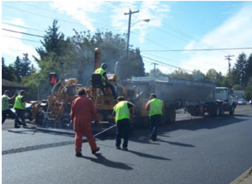
Figure 1 Bureau of Maintenance paving crew applying a pavement overlay
