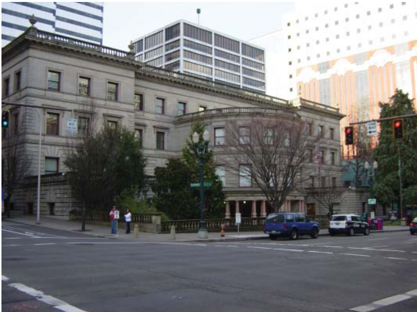
City Hall (Audit Services Division photo)
