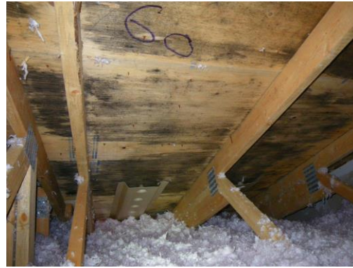
Figure 6: North facing attic roof sheathing for same attic as Figure 13 showing significant fungal growth
