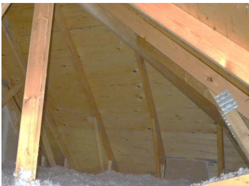
Figure 13: South facing attic roof sheathing for same attic as shown in Figure 14 showing negligible fungal growth
