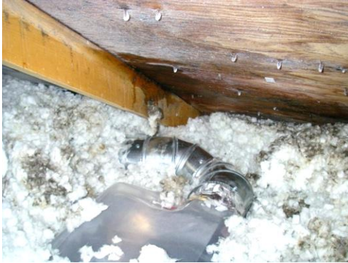
Figure 1: Locally stained and wet sheathing due to condensation (frost) of humid air which is leaking from a poorly sealed bathroom exhaust duct
