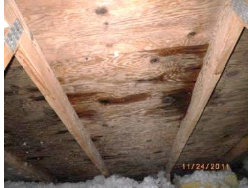
Figure 2: Visibly wet roof sheathing caused by rainwater ingress through the shingles and underlay
