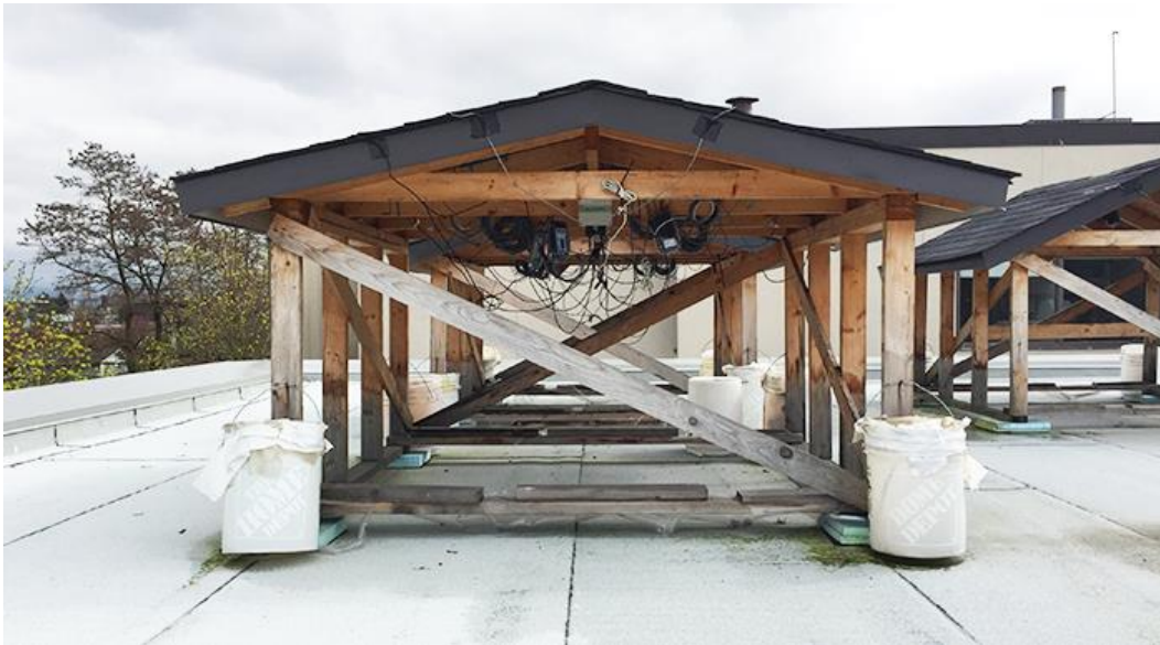
Figure 11: Roof hut decoupled from interior conditions by unrestricted ventilation to the underside of the roof sheathing. Monitoring equipment was installed to measure performance characteristics including sheathing moisture content at various depths, roof surface temperature, sheathing temperature, and ambient temperature and relative humidity.
