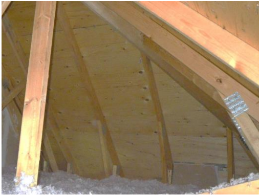
Figure 5: South facing attic roof sheathing for same attic as shown in Figure 14 showing negligible fungal growth
