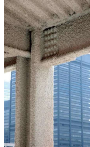
Figure 3 – Steelwork Fire Protected By SFRM Coating System (Photo Courtesy Of GCP Applied Technologies)
