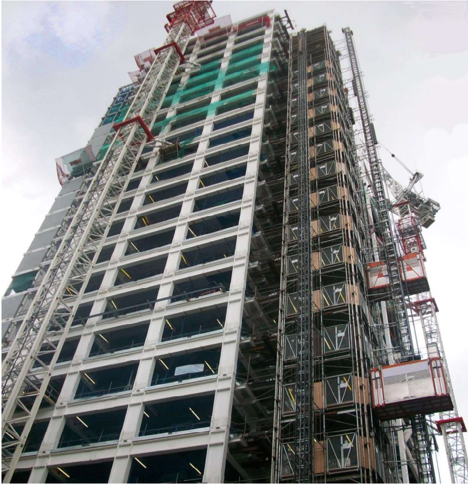
Figure 1 – Steelwork Fire Protected By Intumescent Coating System (Photo Courtesy Of Sherwin-Williams)
