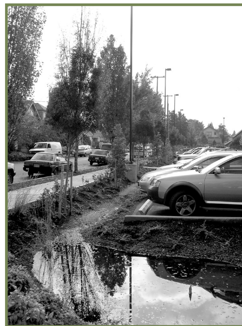
Stormwater swale, recently planted
