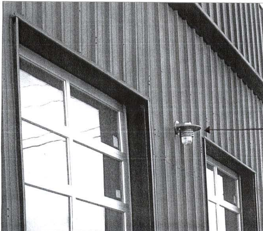
Photo of new garage doors + light fixture (east facade)
