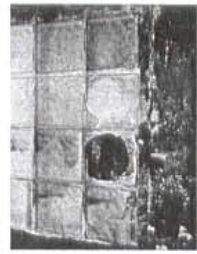
existing glass block
