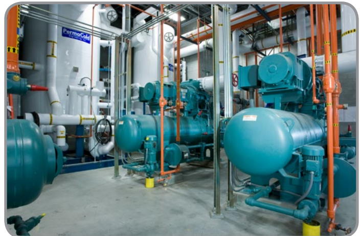
Optimized compressed air systems
