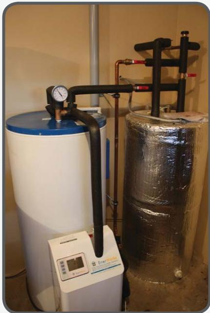
Storage-tank water heaters heat large volumes of water 24 hours-a-day. The standard size tank for a household is 50 gallons. Typical stand-by heat losses are about 15 percent through steel-tank walls and piping. Electric models are resistance-type heaters which use a high amount of energy compared with heat output through two elements. Gas models have the
