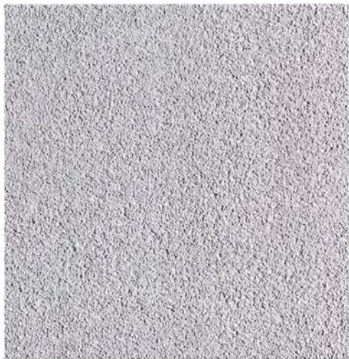
Repaint Existing Painted Stucco
