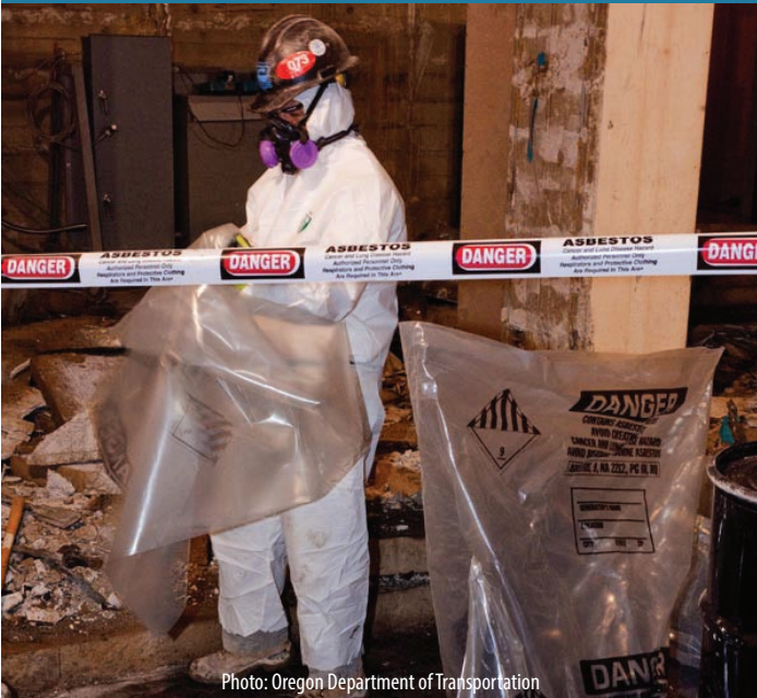
Photo: Oregon Department of Transportation
