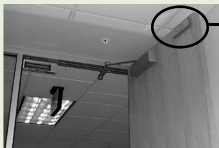
Typical magnetic locking device with required manual release button located near exit
