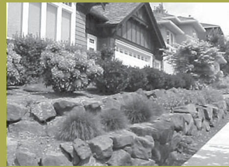
Use tiered planters to stabilize slopes, protect against erosion, and reduce sediment transport.
