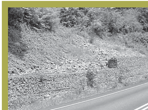
Highly erosive or unstable soils may require reinforced soil retaining systems or armoring.
