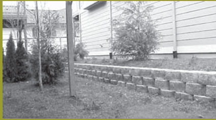
Downspouts, retaining wall and bark dust help with erosion control.
