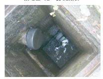
Vortex restrictor installed in a catch basin
