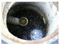
Hanging trap installed in a sedimentation manhole
