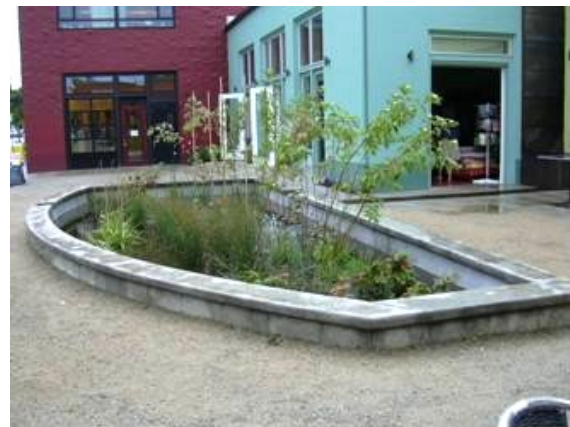
Mississippi Commons After, with Stormwater Infiltration Planter
