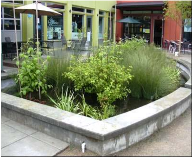
Stormwater Infiltration Planter, looking north
