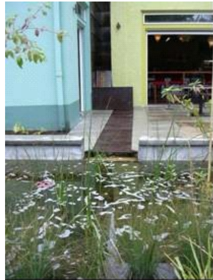
Roof runoff conveyed to the newly vegetated planter
