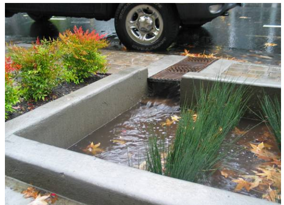
Inlet to Stormwater Street Planter
