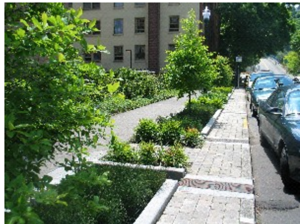
Stormwater Street Planters at SW 12th and Montgomery Portland, Oregon
