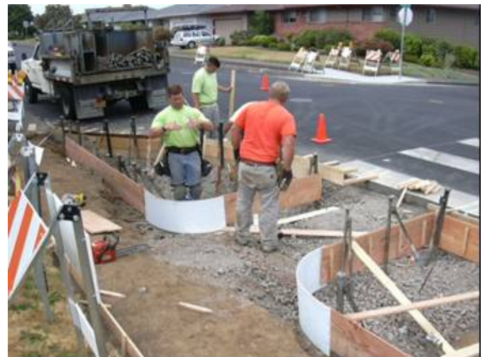
Constructing the stormwater facility; forming the curbs.
