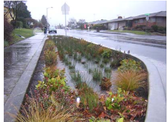
Fremont stormwater curb extension during a rainstorm
