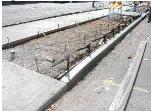
Figure 5: New curb and sidewalk installation
