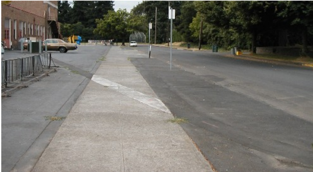
Figure 1: Asphalt parking strip median (middle dark grey areas to right)
