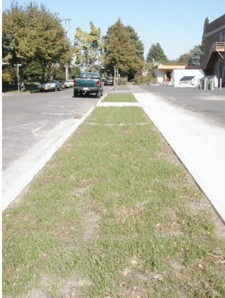
Figure 2: Parking strip medians with grass and concrete pavers for pedestrian access
