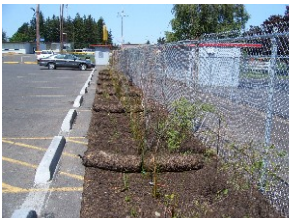
Figure 3 – east swale post construction
