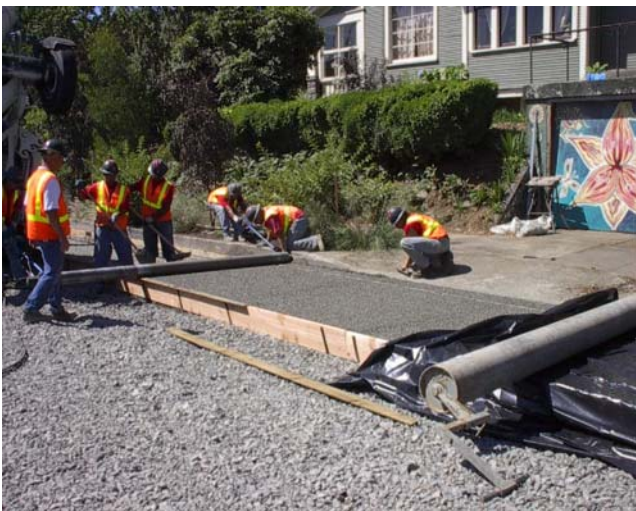
Figure 5: Laying the concrete
