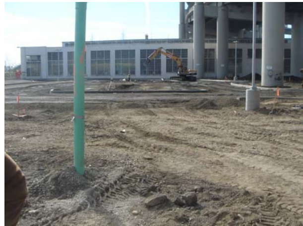
South parking lot looking south during construction
