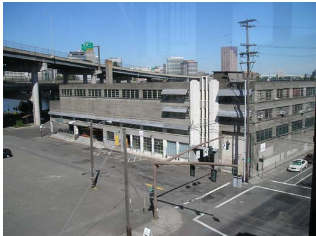
Clay Street from above looking east pre-construction
