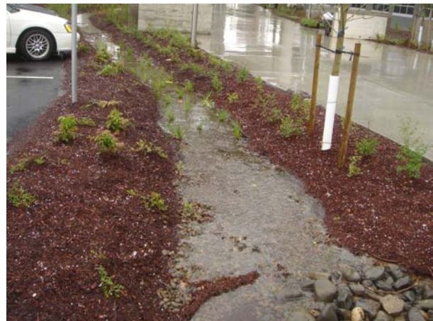
Vegetated infiltration swale along sidewalk
