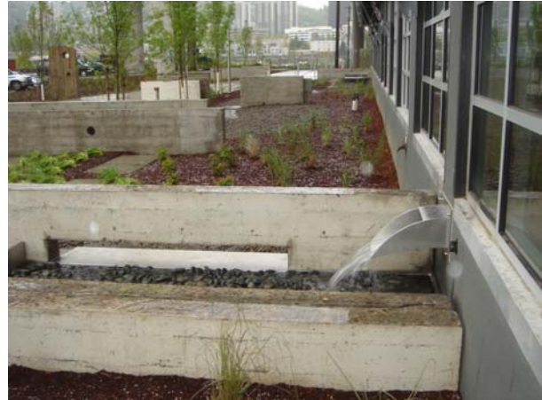
Rain scupper at downspout basin after heavy rain
