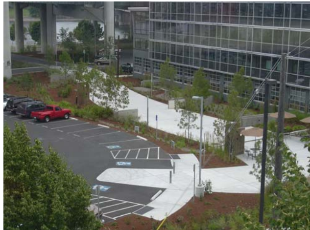
Clay Street from above looking east post-construction
