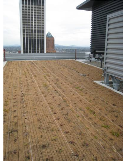
Level 24 Eco-Roof - March 2009
