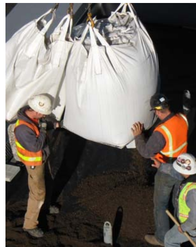
Placing LiteTop® - Dec. 2008
