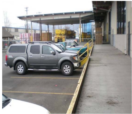
Loading dock before construction
