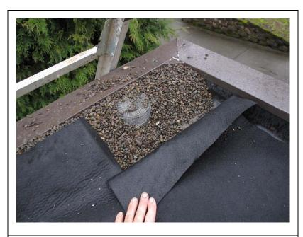
Fig 3. Drain, wire "basket," gravel, and Geotextile detail.
