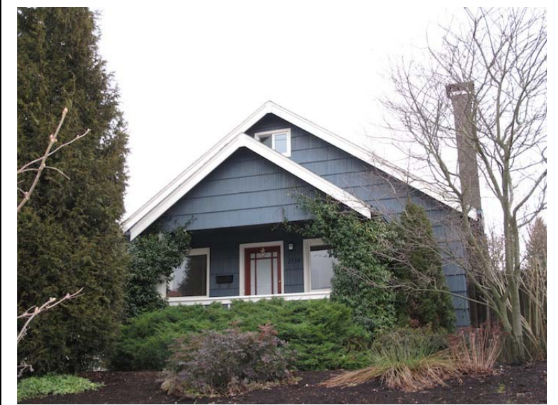
Fig 1. Original porch roof.
