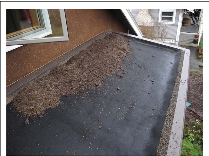
Fig 4 Geotextile on EPDM membrane; soil being added.
