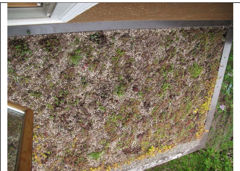
Fig 6. Finished roof with plants.
