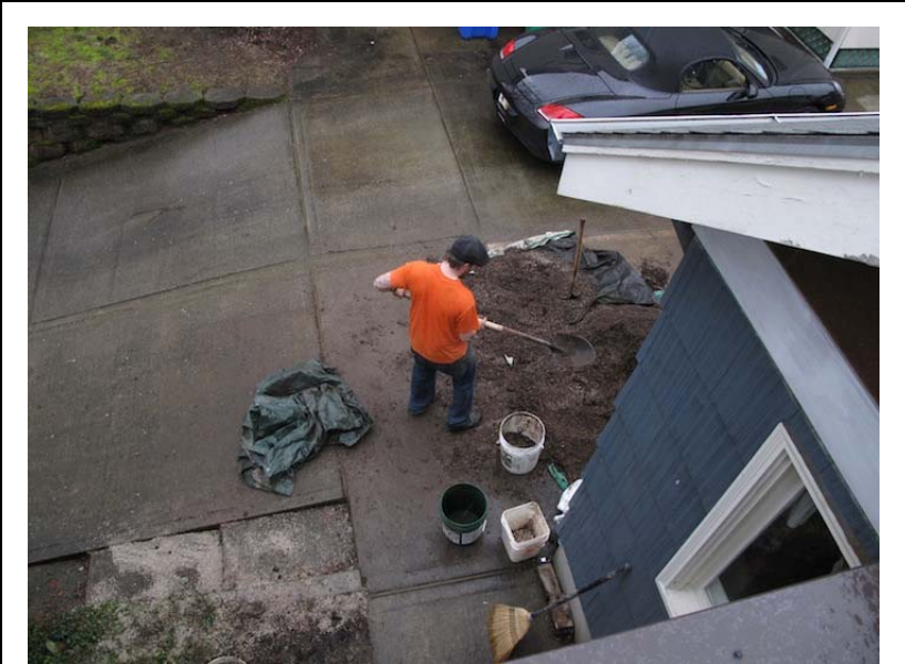
Fig 5. Mixing the soil on the ground.
