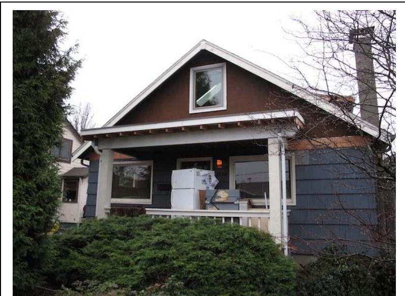
Fig 2. New porch roof.
