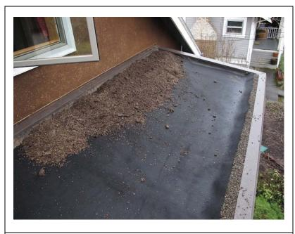
Fig 4Geotextile on EPDM membrane; soil being added.
