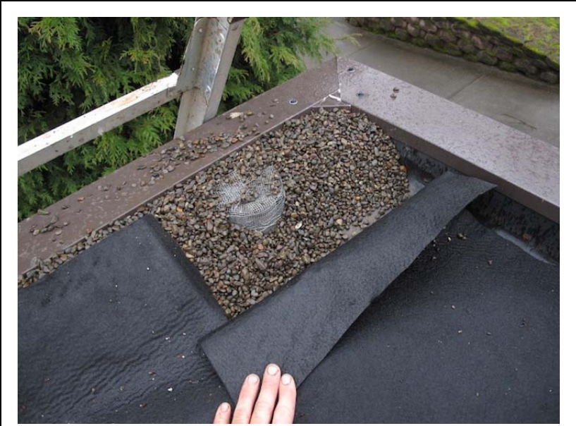
Fig 3. Drain, wire “basket,” gravel, and Geotextile detail.
