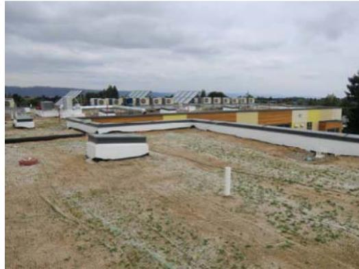
In addition to the ecoroof, the building's parking lot contains stormwater swales designed to filter and retain stormwater. Together with the roof, these elements treat 100 % of the property's stormwater. Additional benefits of the stormwater facilities are the mitigation of the urban heat island effect and providing native habitat.
